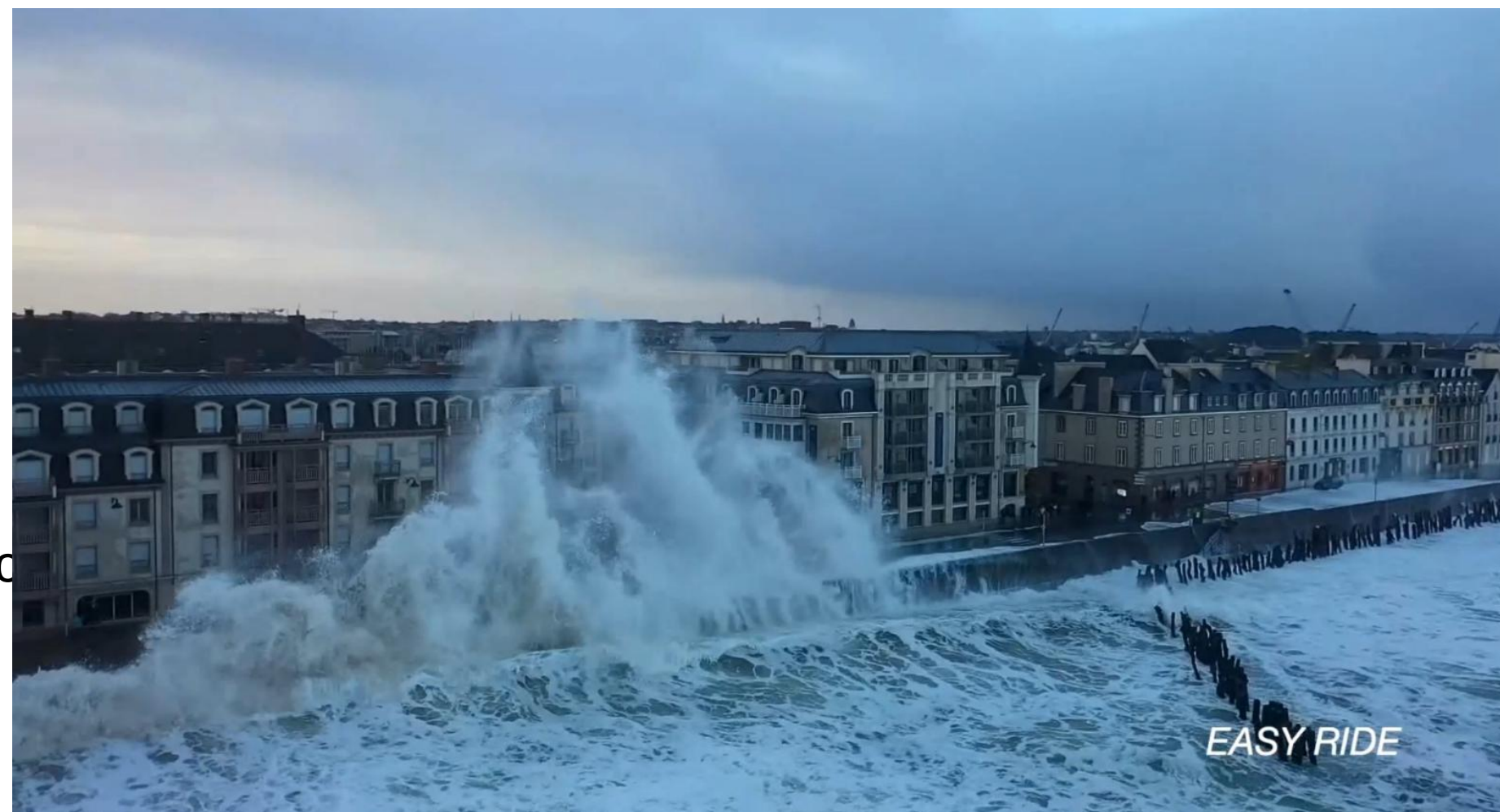
Impact of Storm Ciara (Feb., 2020) on Saint Malo, France (Credit: EasyRideVideos)
